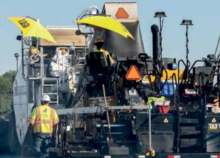
Image: Surfacing work undertaken by Idaho Materials & Construction (IMC), part of our CRH Americas Materials Division on a section of Interstate-84 (I-84) between Nampa and Caldwell, Idaho. Recent harsh winters caused the original surface to deteriorate and IMC completed a fast-track project that included milling out the existing surface, inlaying a base course and overlaying approximately 15km of highway.
