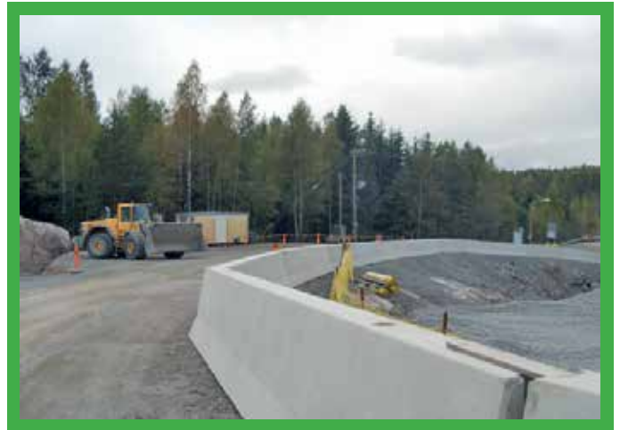
Edge Protection using precast structures.
