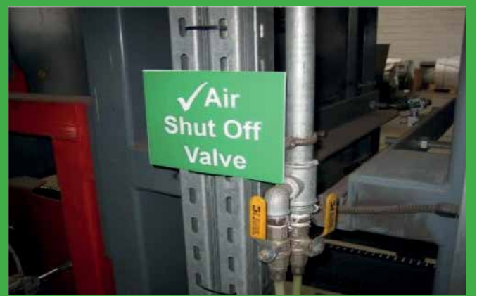
Clearly identified pneumatic isolation point.
