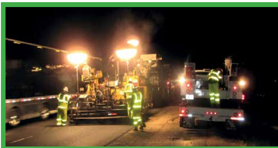
Road-surfacing at night close to live traffic.
