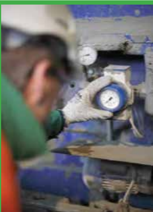
A confirmation check that all residual air has been vented from the system.
