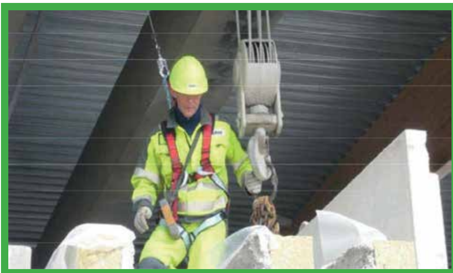
Safe access system for securing and detaching lifting slings
