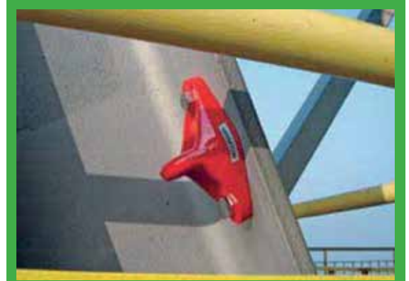
Additional securing hooks for harness use - installed where required.
