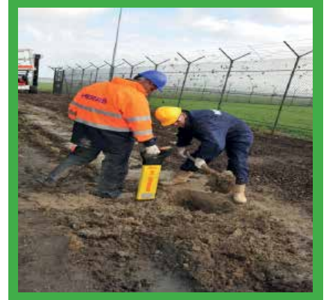
Checking for the presence of underground services prior to the erection of fencing.
